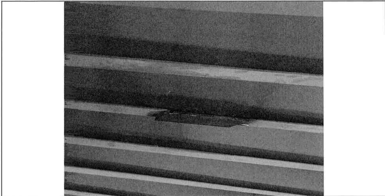
Rafter weld repair
