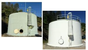
Superior Tank Solutions began the renovation on April 3, 2025, and finished on May 1, 2025. The renovation included installing a new AWWA compliant 30" mushroom vent with a compliant non-corrodible mesh screen to meet EPA and AWWA standards., as well as installed an OSHA compliant roof railing at the roof hatch. They also provided and installed OSHA compliant tie off points on the tank roof next to vents and all hatches.
